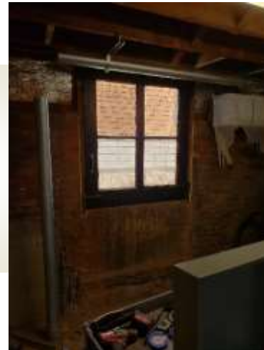
Original Basement Window (to be replaced)
